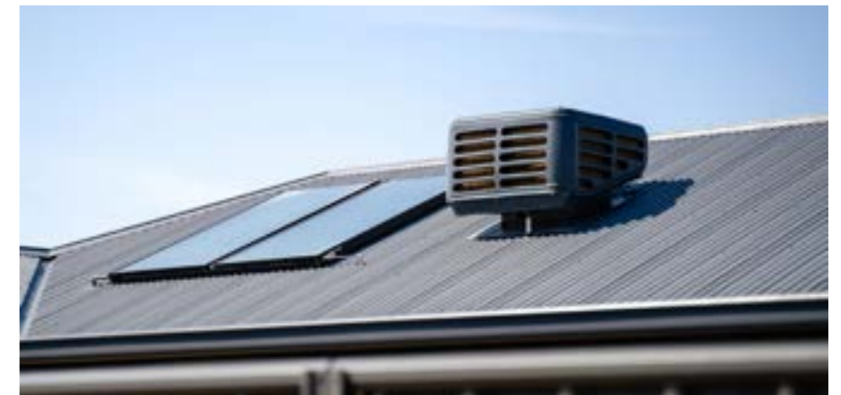
Roof mounted air-conditioning /evaporative cooling units must be towards the rear of the property and below the ridgeline.
